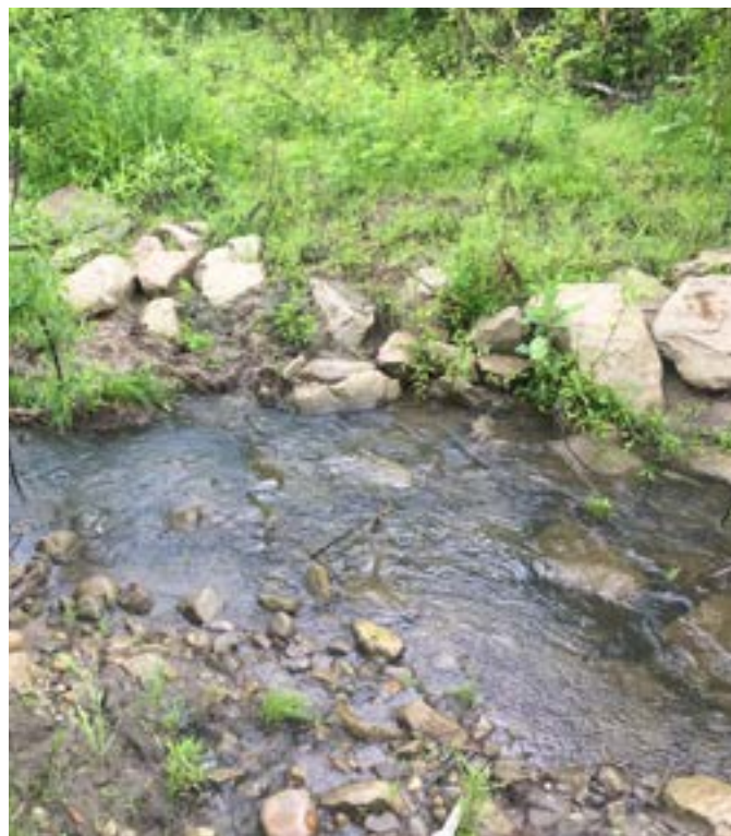
After restoration, installed rock riffles increase connection to natural floodplain, slowing waters down and filtering out sediments. Photo credit: Chagrin River Watershed Partners
