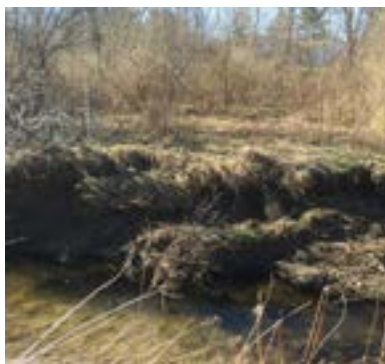
Before restoration, heavy erosion of the streambank offered no floodplain connection, causing silt to wash downstream. Photo credit: Chagrin River Watershed Partners
